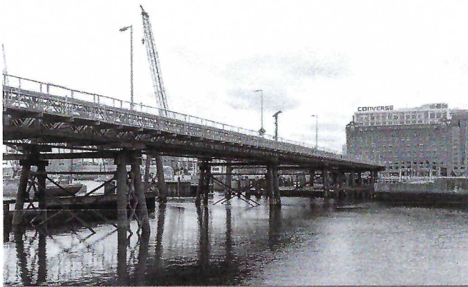
View of the temporary bridge structure under construction. Photo: December 2020
